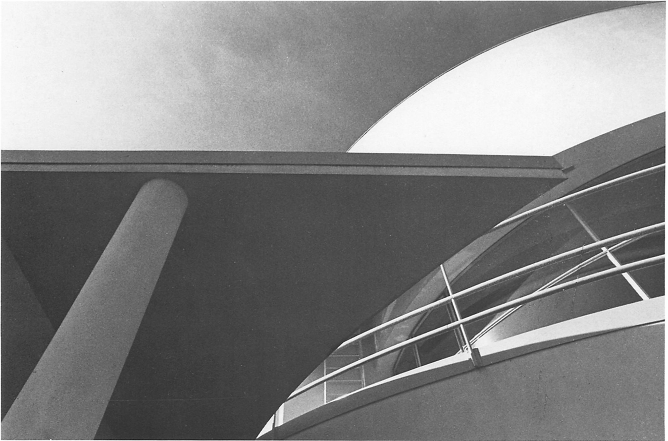
18. View of canopy and ramp to third level
